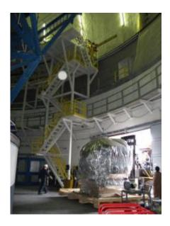
The carefully wrapped MOSFIRE instrument is forklifted into the ground-floor of the Keck I Telescope dome. In coming weeks it will be lifted to an upper deck and prepared for installation on the telescope itself. Credit: W. M. Keck Observatory
