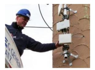
A researcher positions a WiBACK network antenna. Credit: Fraunhofer FOKUS
