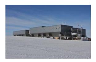
Elevated new Amundsen-Scott South Pole station is built on the 9000 ft. thick polar ice sheet. Credit: NSF
