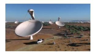
An artist's impression released by the SPDO shows dishes of the future Square Kilometre Array radio telescope. Dishes will form a substantial part of the SKA; around 3000 dishes, each 15 m in diameter, are currently planned. South Africa is well-placed to host the world's largest telescope because it would cost cheaper, according to the deputy science minister.
