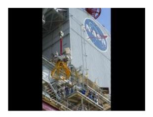
Stennis Space Center engineers and technicians watch as the J-2X powerpack is hoisted into place in the A-1 test stand Dec. 5. Credit: NASA/SSC
