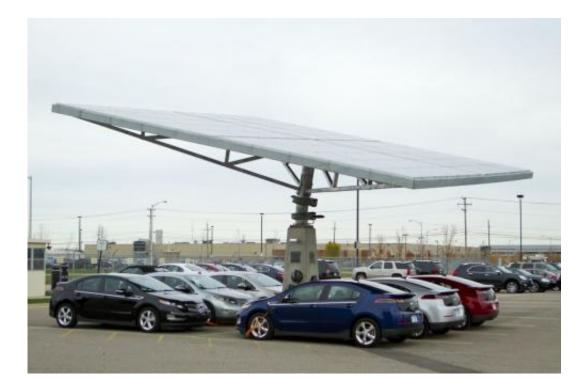
General Motors is introducing a solar charging canopy that moves with the sun. The Tracking Solar Tree is located at GM Company Vehicle Operations.
