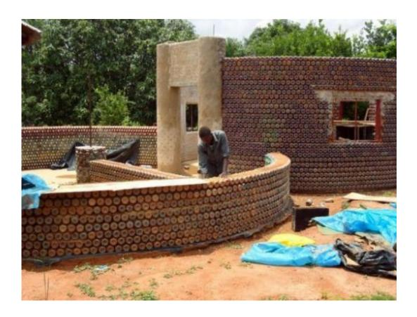
A man builds a wall with plastic bottles in the village of Sabon Yelwa. A group of activists have come up with a plan to build a house using bottles, providing what they say is an environmentally smart way to tackle the housing shortage problem in Nigeria.
