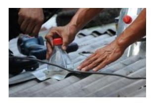
Soldiers install solar light bottles on a roof in a Manila shanty town. The idea is simple - fill discarded soft drink bottles with water, place them in roofs and allow the refracted light to brighten homes during the day.
