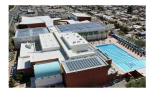
The Solar Thermal Array installed on top of the UA's recreation center (in the background) has an estimated annual production equivalent of almost 2 million kilowatt-hours and is expected to reduce greenhouse gas emissions by 1,317 metric tons per year. It is the latest addition in a portfolio of innovations promoting energy efficiency and sustainability on the UA campus. (Photo: Ameresco Southwest)
