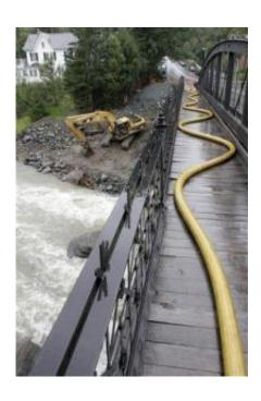
A hose carries the town water supply over the Ottauquechee River, replacing a water main running under the river which was washed away on Wednesday, Sept. 7, 2011 in Woodstock, Vt. Drinking water supplies in Vermont suffered damages in flooding from Tropical Storm Irene. Some communities remain under boil water orders and private well owners are being urged to have their tests for contaminants. (AP Photo/Toby Talbot)
