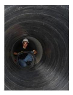
In the innovative PipeMedic repair system developed by University of Arizona civil engineering professor Mo Ehsani, the carbon fabrics of any design (up to a width of 60 inches) are saturated with the resin and run through a special press; the result is a solid "super" laminate with a thickness that can be set from 0.02 to 0.08 inches. Credit: PipeMedic.com
