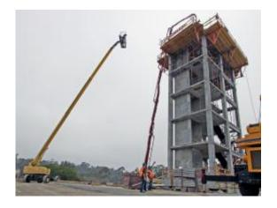
Two graduate students look on as construction crews pour the roof slab on a fivestory building at Englekirk Center. The building will be outfitted to test nonstructural components, including a working elevator, stairs, a sprinkler system and medical equipment.
