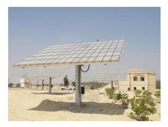
The concentrating photovoltaic modules in Egypt are precisely aligned to the sun. They supply power to irrigate wheat fields. (© Fraunhofer ISE)
