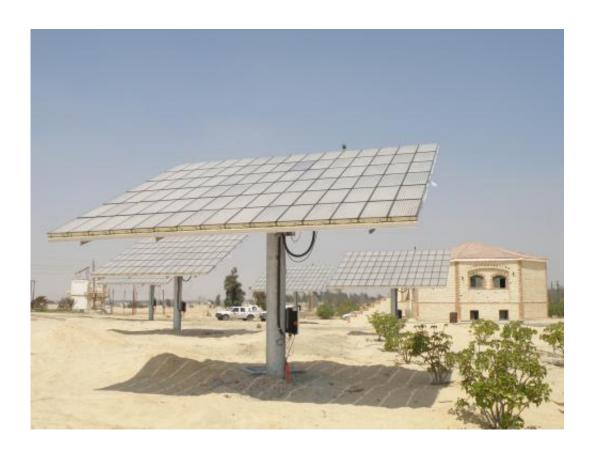
The concentrating photovoltaic modules in Egypt are precisely aligned to the sun. They supply power to irrigate wheat fields. (© Fraunhofer ISE)
