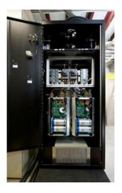
NREL's 50 kW Power Blocks will be housed in inverter cabinets as shown in this photo. The power block rests above the air-intake blower and below the AC and DC protection devices, an accessory rack and air-out fans. The entire package is about 6 feet high,  $2\frac{1}{2}$  feet wide and  $2\frac{1}{2}$  feet deep. Credit: Dennis Schroeder
