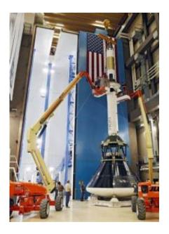
Engineers attach a collar to the escape vehicle on the Orion spacecraft at the Lockheed Martin facility in Denver on Friday, Aug. 12, 2011. They will use it to move the assembled craft to the testing chamber at left where it will be submitted to vibration testing. (AP Photo/Ed Andrieski)
