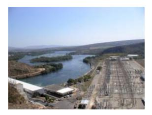
Located on the middle of the Rio Grande, the UHE FURNAS reservoir is one of the largest in Brazil. It impounds the Grande River and has a capacity of 22,590,000,000 m3 and a surface area of 1,473 km2. Credit: Fábio Roland
