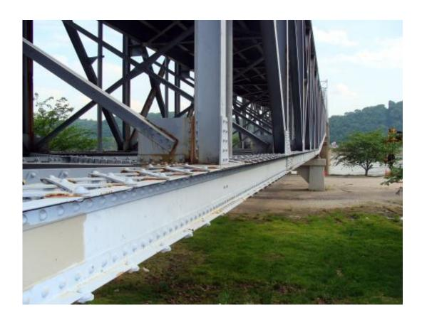
A Purdue civil engineer is taking advantage of the demolition of a bridge spanning the Ohio River to learn more about how bridges collapse in an attempt to reduce the annual cost of inspecting large spans. He will purposely damage this approach span leading to the Milton-Madison Bridge in southern Indiana, which is being demolished in stages. (Purdue School of Civil Engineering photo/Ryan Sherman)
