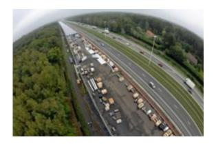
Workers install solar panels for the Hybrid solar lighting (HSL) tunnel in Brasschaat, Belgium in 2010. High-speed international trains linking Paris and Amsterdam became the first in Europe to use electricity generated by solar panels installed in a tunnel on the line.
