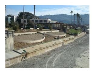
Storm water that falls on the grounds of Scripps Institution of Oceanography passes through an innovative water-pollution-control system, including these two inconspicuous semicircular 'media filters' to remove pollutants before the water enters the ocean. Credit: Kimberly McConnell/UC San Diego
