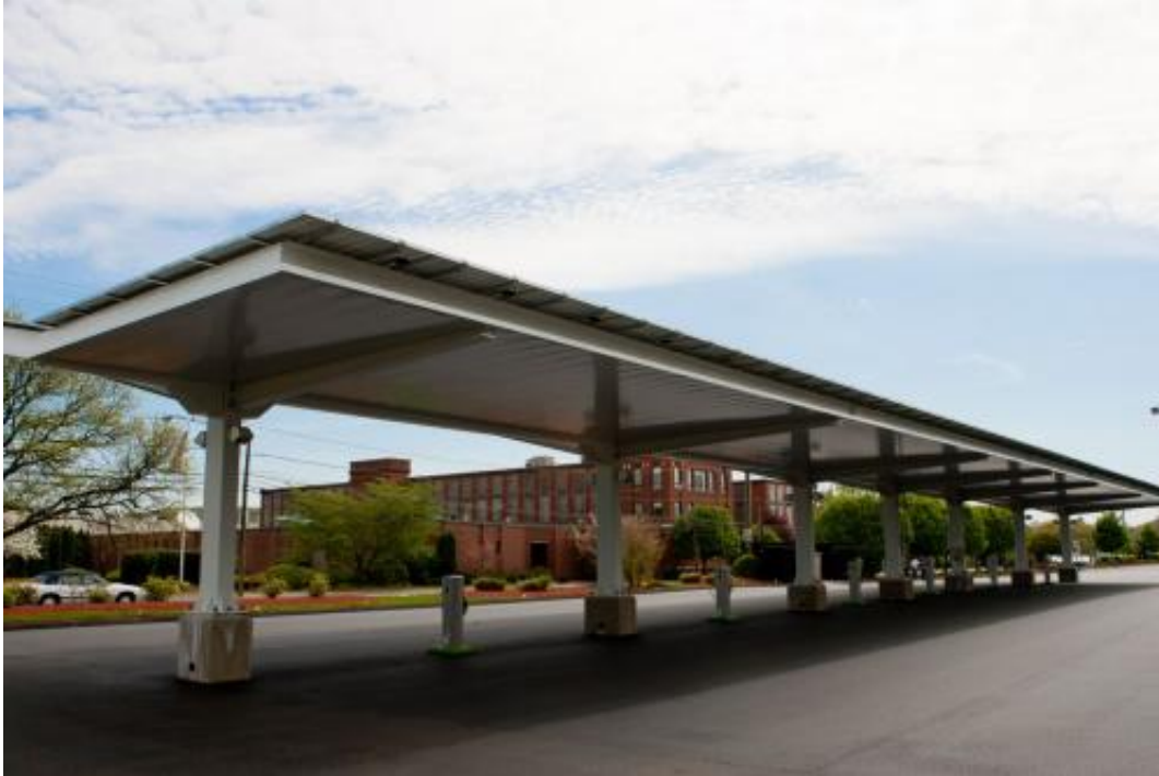
GE EV Solar Carport in Plainville, CT
