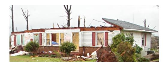
The roof blew off this house during the massive April, 2011, tornadoes in the South due in part to inadequate connections between the roof trusses and the sidewalls. (Photo courtesy of Oregon State University)
