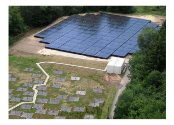
The Lofar station Effelsberg. In the foreground, the dipole field for low frequencies (30 to 80 megahertz, corresponding to between 3.8 and 10-metre wavelength); at the back, the "tile field" for higher frequencies (110 to 240 megahertz or 1.3 to 2.7-metre wavelength. Credit: Max Planck Institute for Radio Astronomy / Wolfgang Reich
