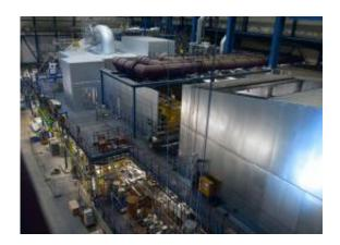
A new Siemens gas turbine operated in a combined cycle with a steam turbine in Irsching, Bavaria, has set a world record for efficiency, making it an outstanding example of green technology. The net efficiency of 60.75 percent achieved during the test run even surpassed the target value of 60 percent; the previous generation of the turbine had an efficiency of 58.5 percent. The new turbine is designed to generate 400 megawatts (MW) alone and 600 MW when combined with a steam turbine.
