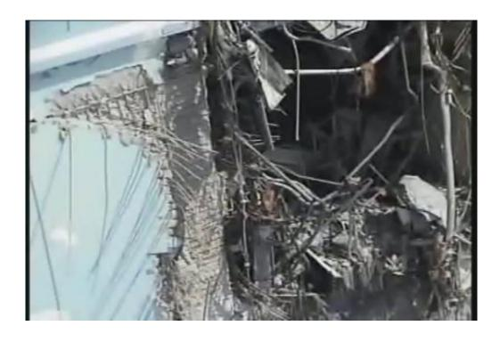
This handout picture taken by a Tokyo Electric Power Co remote controlled drone on Friday and released on Sunday shows the wrecked south side wall of the fourth reactor building at TEPCO's Fukushima No.1 nuclear power plant.
