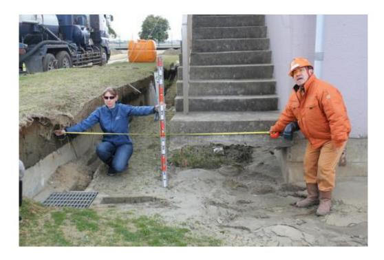
Liquefaction induced by the recent earthquake in Japan caused nearly three feet of settlement at this water purification plant that serves 19,000 people, breaking pipes and flooding underground structures. Measuring the damage are Jennifer Donohue, a member of the Geotechnical Extreme Events Reconnaissance team with Geosyntec Consultants, and an engineer from the Wanigawa Water Purification Plant. (Photo by Scott Ashford, courtesy of Oregon State University)
