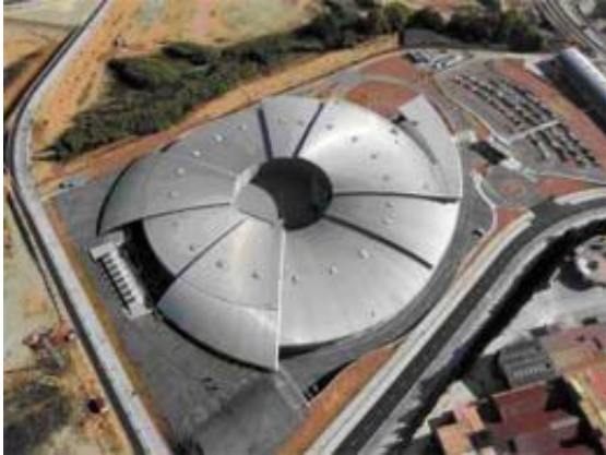
ALBA Synchrotron Light Facility
