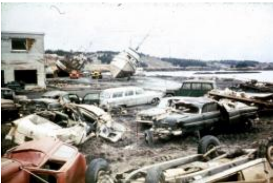
Tsunami damage along the waterfront of Kodiak, Alaska, after the 1964
