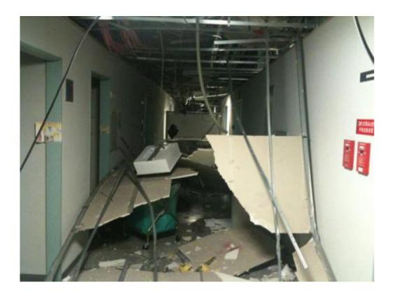
This photo shows some of the damage to the Tsukuba Space Center in Tsukuba, Japan, the main space center for the country's JAXA agency, from the 8.9-magnitude earthquake that struck on March 11, 2011. Credit: collectSPACE.com
