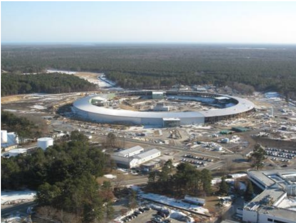
NSLS-II construction site
