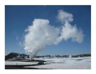
This is a view of the exploratory geothermal well during flow testing. Credit: Bjarni Palssen.
