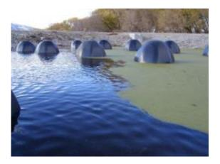
Poo-Gloos -- inexpensive devices to extend the lifespan of sewage lagoons for towns and small cities outgrowing their waste-treatment facilities -- are half submerged as officials fill this sewage lagoon in Wellsville, Utah. The iglooshaped devices are submerged when operating, and a new study shows they remove organic waste and other pollutants from sewage just as well as much more expensive mechanical sewage-treatment plants. Credit: Waste Compliance Systems Inc.
