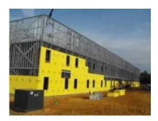
Cold-formed steel has become a popular construction material for commercial and industrial buildings, but a key question remains: How can these structures be designed so that they are most likely to remain intact in a major earthquake?
