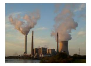
60 percent of the energy used in large-scale power plants is lost as waste heat through the cooling tower. Credit: Fraunhofer UMSICHT
