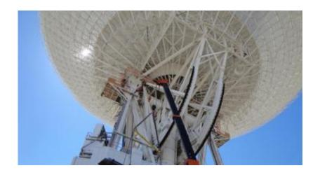
Under the unflinching summer sun, workers at NASA's Deep Space Network complex in Goldstone, Calif., use a crane to lift a runner segment that is part of major surgery on a giant, 70-meter-wide antenna.
