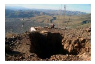
View of a collapsed section at the Cerro Rico mountain - one of the world's biggest silver deposits, in Potosi. The five-century exploitation of the deposit which left more than 600 pitheads and 90 km of tunnels is causing severe subsidences and landslides.
