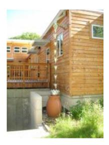
A chain of rainflowers guides rainwater from the lower roof to a rain barrel, which is tapped to water landscaping. Credit: Ralph Bicknese/Hellmuth + Bicknese
