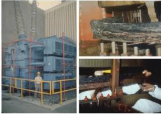
Permanent damage to the Salem New Jersey Nuclear Plant GSU Transformer caused by the March 13, 1989 geomagnetic storm. Photos courtesy of PSE&G.
