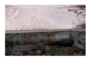
An aerial view of a damaged section of a broken dyke of a reservoir that contained red mud of an alumina factory near Ajka, 156 kms southwest of Budapest, Hungary, Wednesday, Oct. 6, 2010. The dyke broke on Monday, and over one million cubic meters of the poisonous chemical sludge inundated three villages, killing an unknown number of persons and injuring over hundred. Three people are unaccounted for and hundreds of families have been evacuated. (AP Photo/MTI, Sandor H. Szabo)
