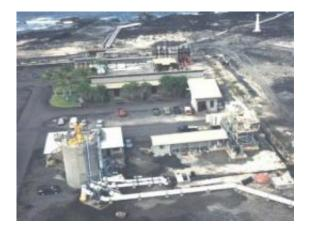
An example of early OTEC field work in Hawaii: aerial view of the land-based experimental open-cycle OTEC plant that operated between 1993 and 1998 on the Big Island. The facility still holds the world record for OTEC power production, with turbo-generator output exceeding 250 kW and more than 100 kW of net power exported to the grid. Credit: Luis Vega
