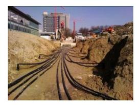
The ground heat probes are combined together by manifolds which then lead into the ETH Zurich ring system. (Photo: Amstein + Walthert AG)
