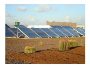
Fraunhofer ISE intends to contribute to the development of solar-powered water desalination plants such as the one shown here, in Gran Canaria. (© Fraunhofer ISE)
