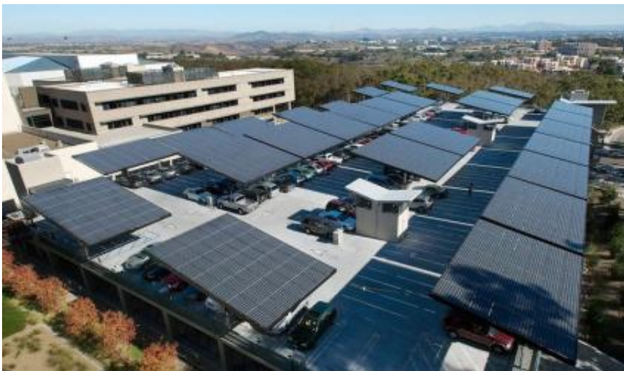
Hopkins Parking Structure, a recent addition to the UC San Diego campus.
