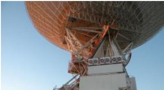
As the sun sets on July 8, 2010, workers prepare to pour new epoxy grout for the hydrostatic bearing assembly of the giant "Mars antenna" at NASA's Deep Space Network communications site in Goldstone, Calif.
