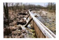
Palisade timber dam lining a hydrological compartment, where the water table was raised. Photo credit: Wilco Verberk.
