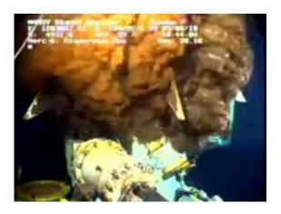
This still image from a live BP video feed shows oil gushing from a leaking BP oil well-pipe in the Gulf of Mexico, June 5. Engineers searched for ways to capture more oil flowing from a raptured well in the Gulf of Mexico Sunday after energy giant BP said a cap was currently catching around 10,000 barrels a day.
