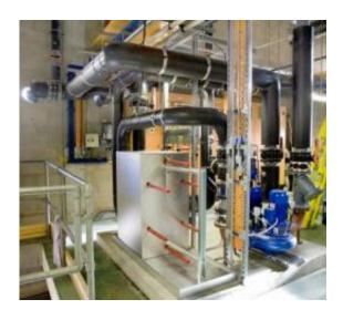
The heat exchanger is a key part of the seawater cooling system at the National Oceanography Center in Southampton. Credit: NOC
