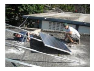
Students at Rensselaer Polytechnic Institute designed, built, and installed a 2.4-kilowatt solar power system on the roof of a school Lascahobas, Haiti. The system is robust enough to power 10 tablet laptop computers donated by Rensselaer, plus additional laptops the school and other nearby schools received from the One Laptop Per Child program. Credit: Rensselaer/Alex Worcester
