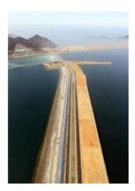
This bird eye view taken on April 20, shows the 33.9 kilometer Saemangeum seawall in Gunsan, some 200 kilometers south of Seoul. S.Korea on April 27 formally marked completion of the world's longest seawall, the first step in a massive project aimed at reclaiming the ocean for industry, tourism and agriculture by 2020.
