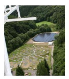
A LOFAR station. This show the 'tiles' of the Low Band Array and the High Band Array at the Eiffelsberg LOFAR station outside Bonn in Germany. The white structures at the upper left are the Bonn 100-metre radio telescope from which this photograph was taken. Image credit: ASTRON/ MPIfR
