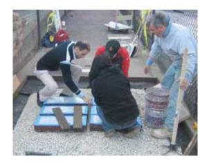
Civil and environmental engineering assistant professor Naji Khoury, left, supervises the installation of six slabs of porous Plastisoil in a walkway outside the College of Engineering. Assisting are two undergraduate engineering students and a contractor, right.
